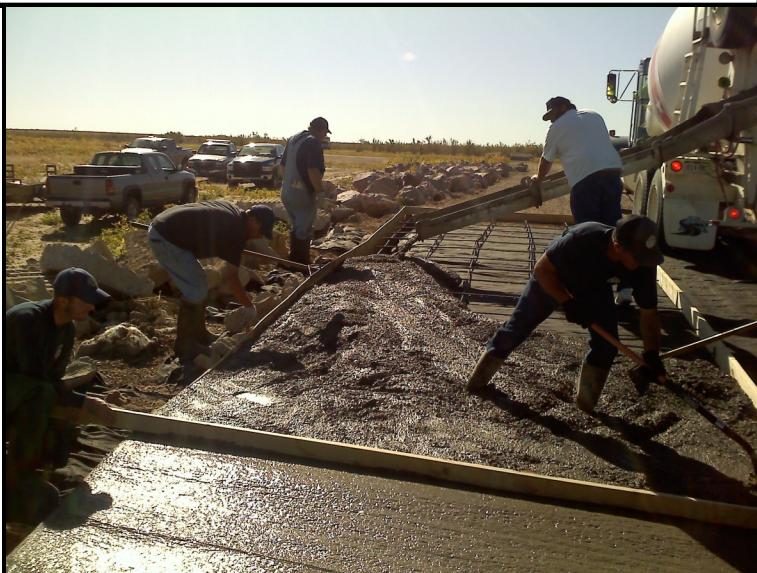
Low Water Ramp Renovation at Adobe Creek Res. 10/11
